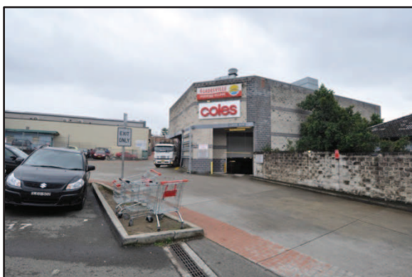
Figure 17. View of the Gladesville Shopping Village from the south, towards the entrance of the basement car park. (Source: Heritage21, July 2012).
